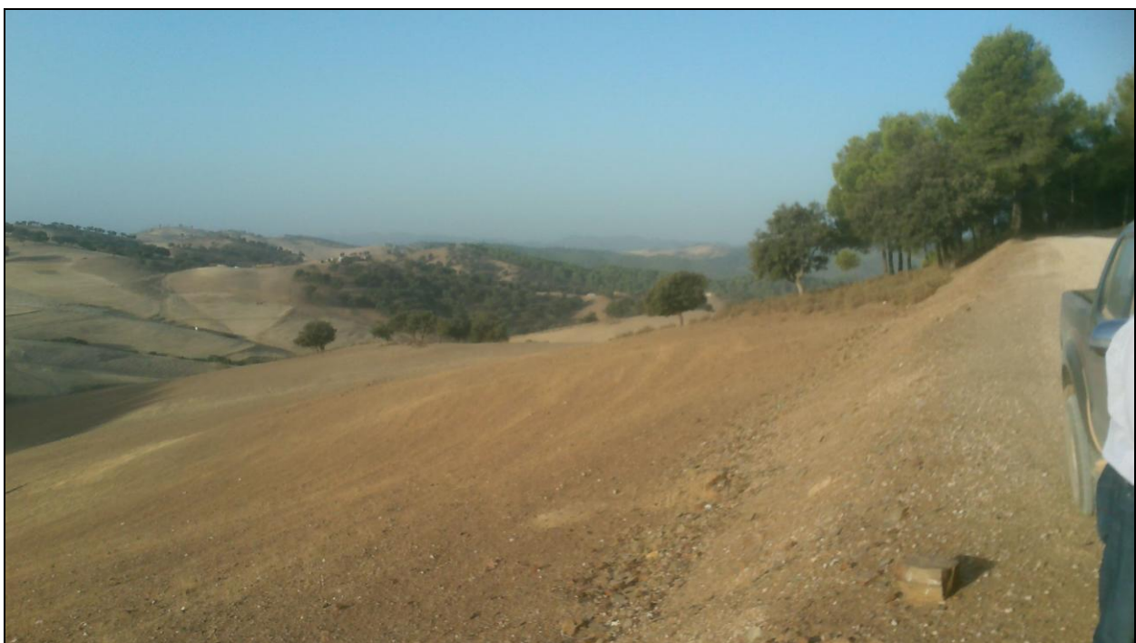
Figure 2 – Proposed area for the processing facilities at Achmmach (already with good road access)
